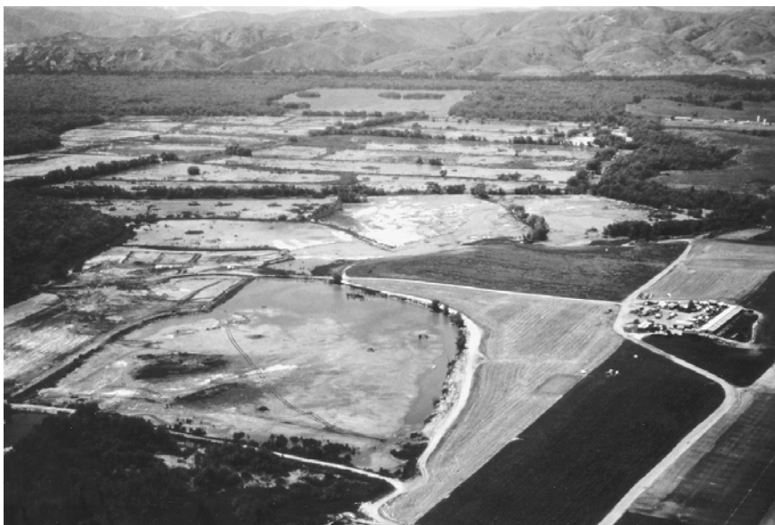
FIGURE 2.1 Aerial view of a full-scale phytoremediation wetland: Prado Wetland, Riverside, CA. This 200-ha (500-acre) wetland removes nitrate from the Santa Ana River which contains more than the 10 mg/l nitrate-N allowed by public health standards. Open water areas alternate with cattail, bulrush, grasses, and duckweed to provide carbon of variable biological lability for bacterial denitrification.
